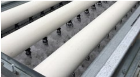
Reduce Downtime by Inspecting the Nozzles While the Unit is in Operation
